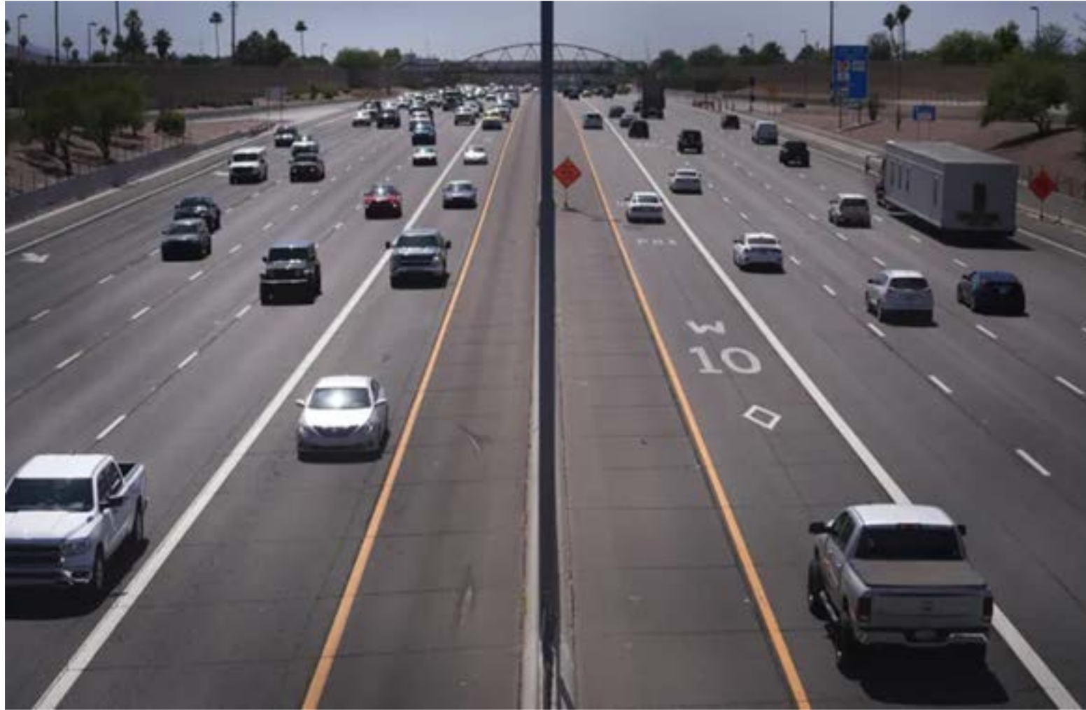
MnDOT Design options 9: Expanded Freeway A Expand the Highway 8-10 Lanes, including MnPass lanes
