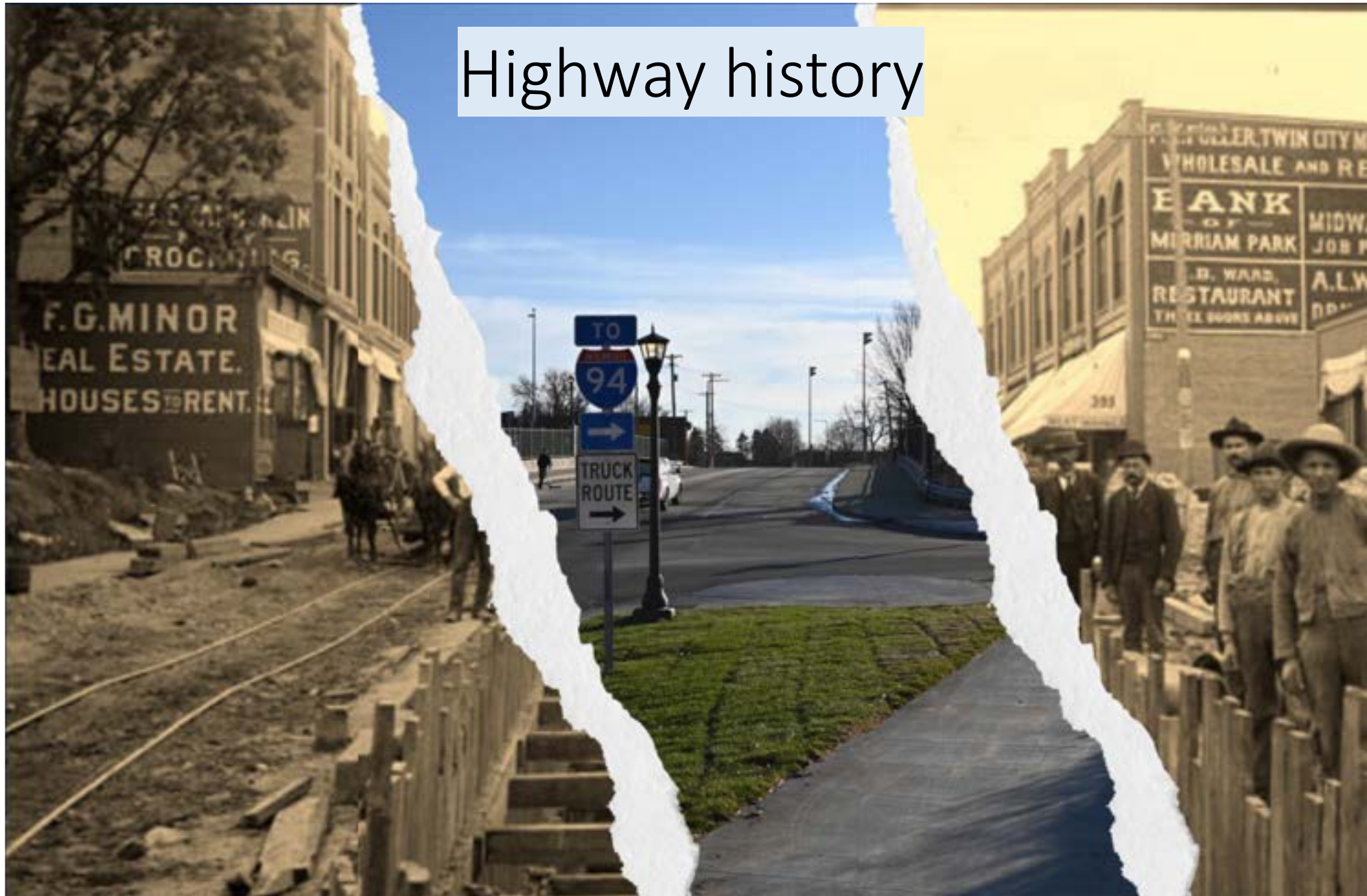
Before and After - Major commercial area at Prior and old St Anthony Avenue
